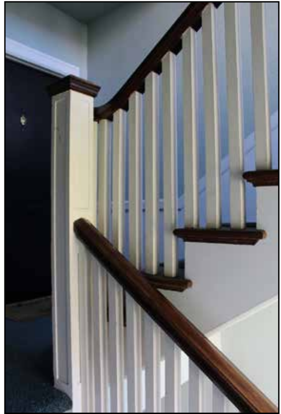
Fig 42. Typical apartment stair off courtyard.
