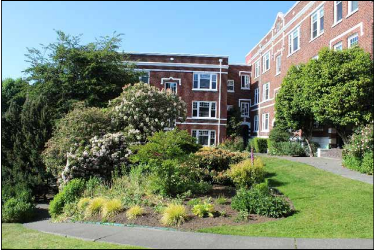
Fig 32. View of garden, concrete paths, and northeast corner of courtyard.
