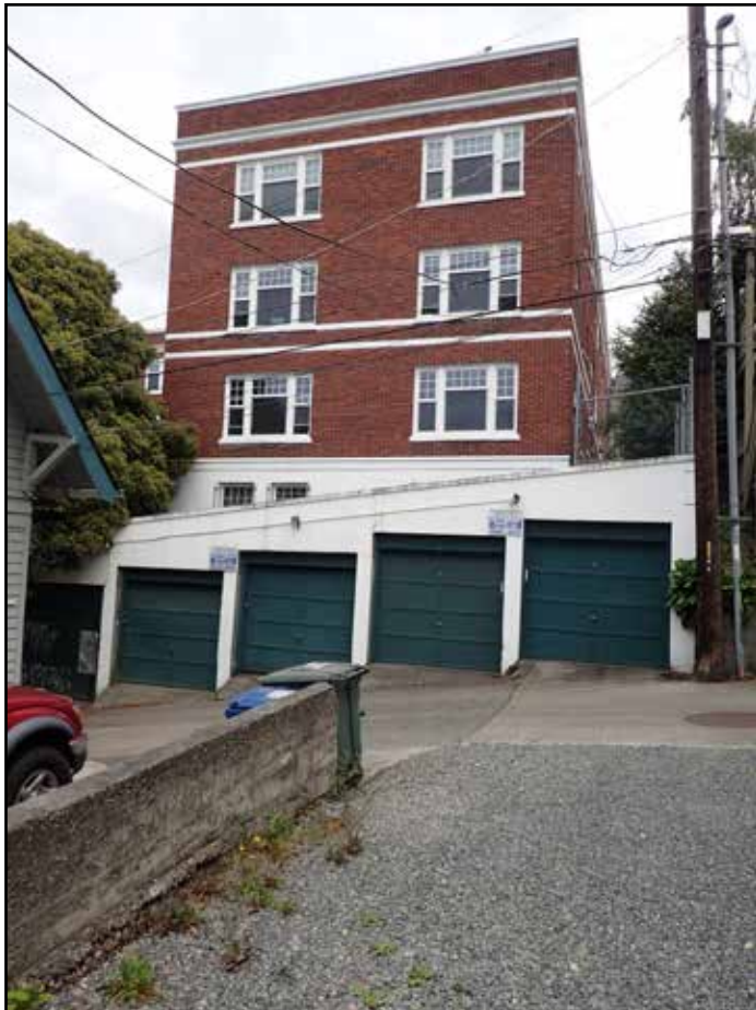
Fig 38. South end of garage, with south wing of Roy Vue above, looking east.
