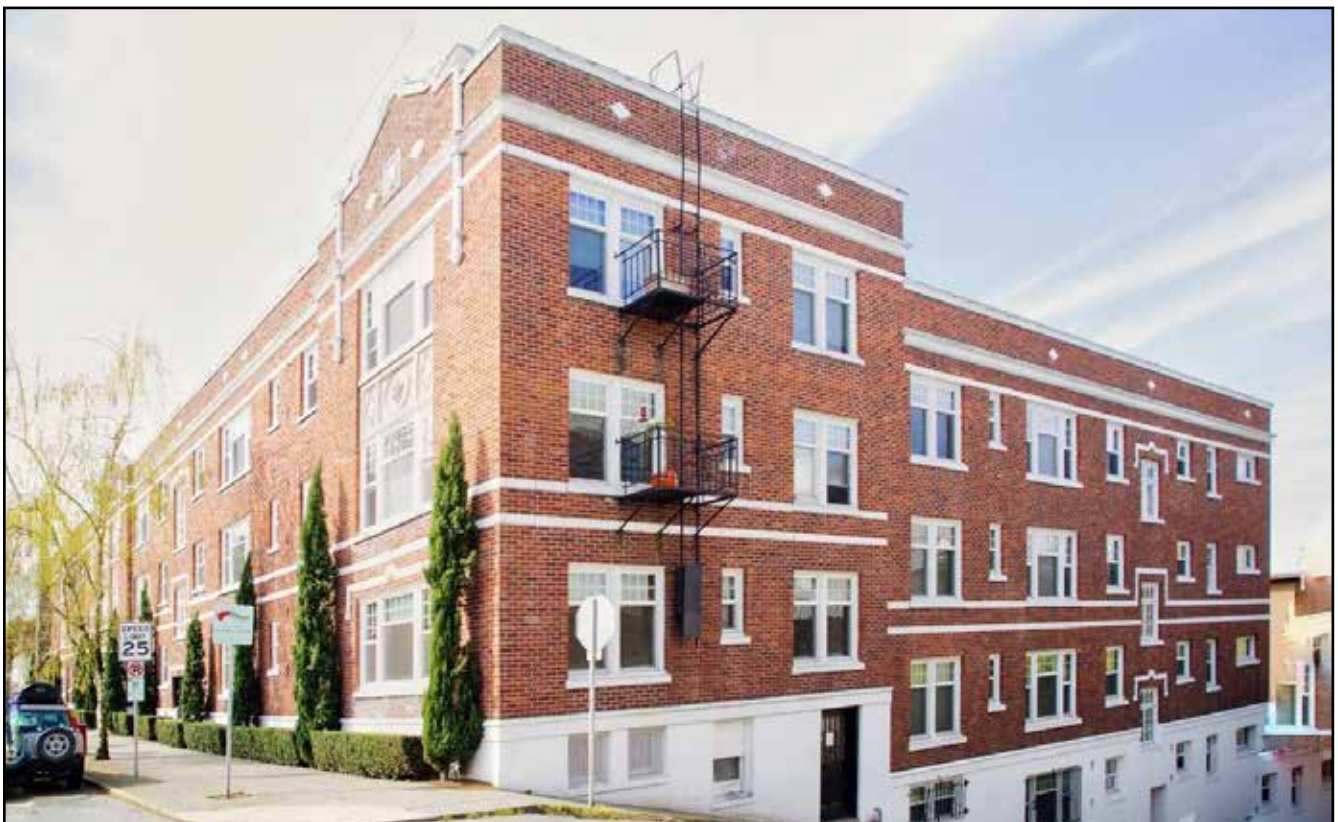
Fig 27. East (primary) and north (side) facades, looking southwest. Source: Save the Roy Vue
