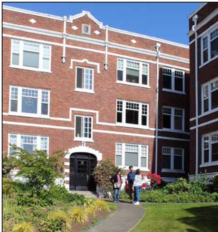
Fig 33. View of garden, concrete path, and southeast corner of courtyard.
