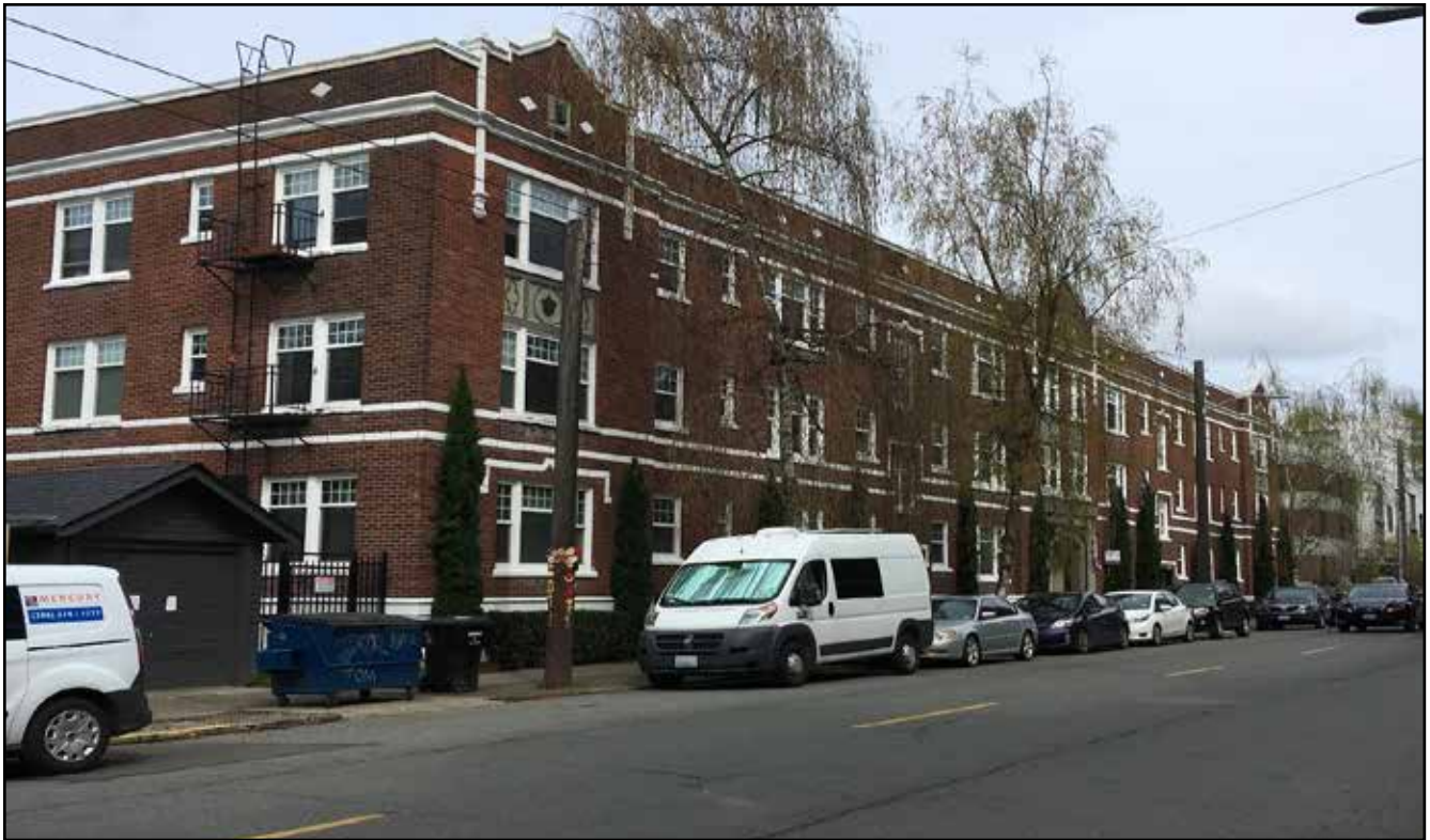
Fig 26. Partial south (side) and east (primary) facades, looking northwest.
