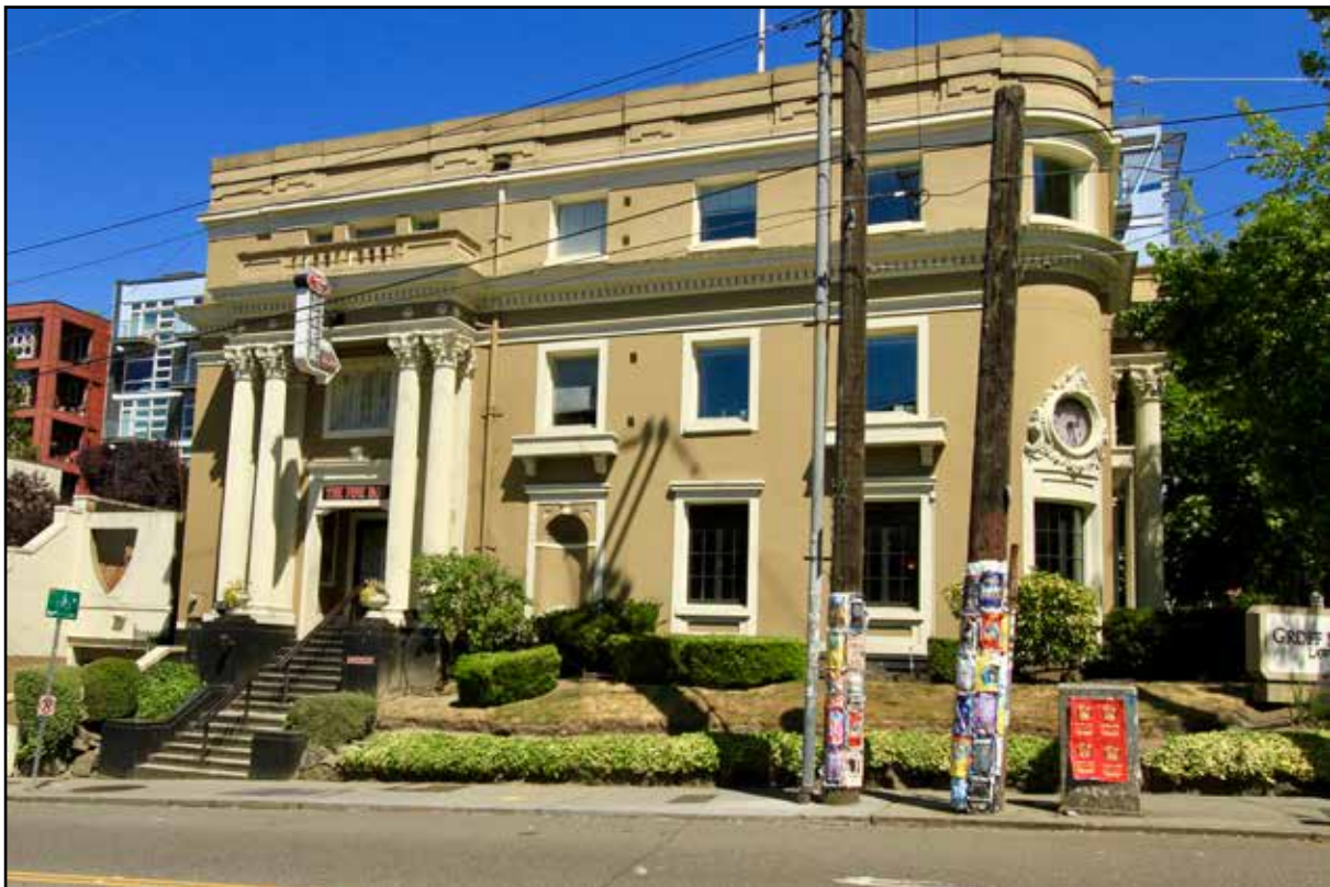
Fig 55. Butterworth Mortuary, 1600 Melrose Ave. (1922; Charles Haynes, architect)
