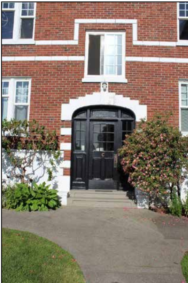
Fig 40. Original wood apartment entry door with side lights off courtyard.
