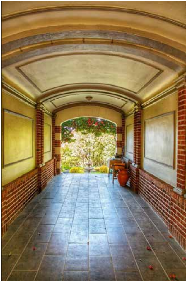
Fig 30. View west into the courtyard through arcade. Source: Save the Roy Vue
