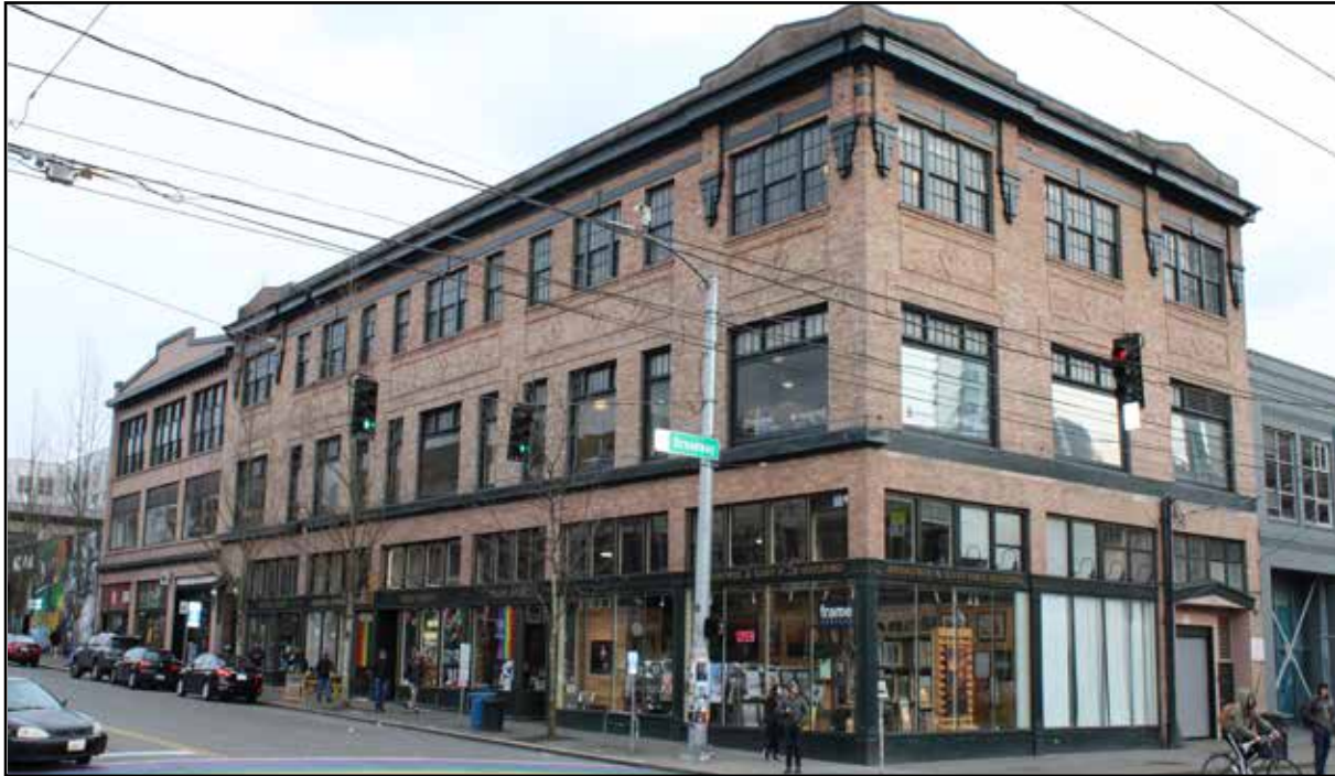
Fig 54. Tyson Oldsmobile Company, 905 E. Pike St. (1912; Charles Haynes, architect)
