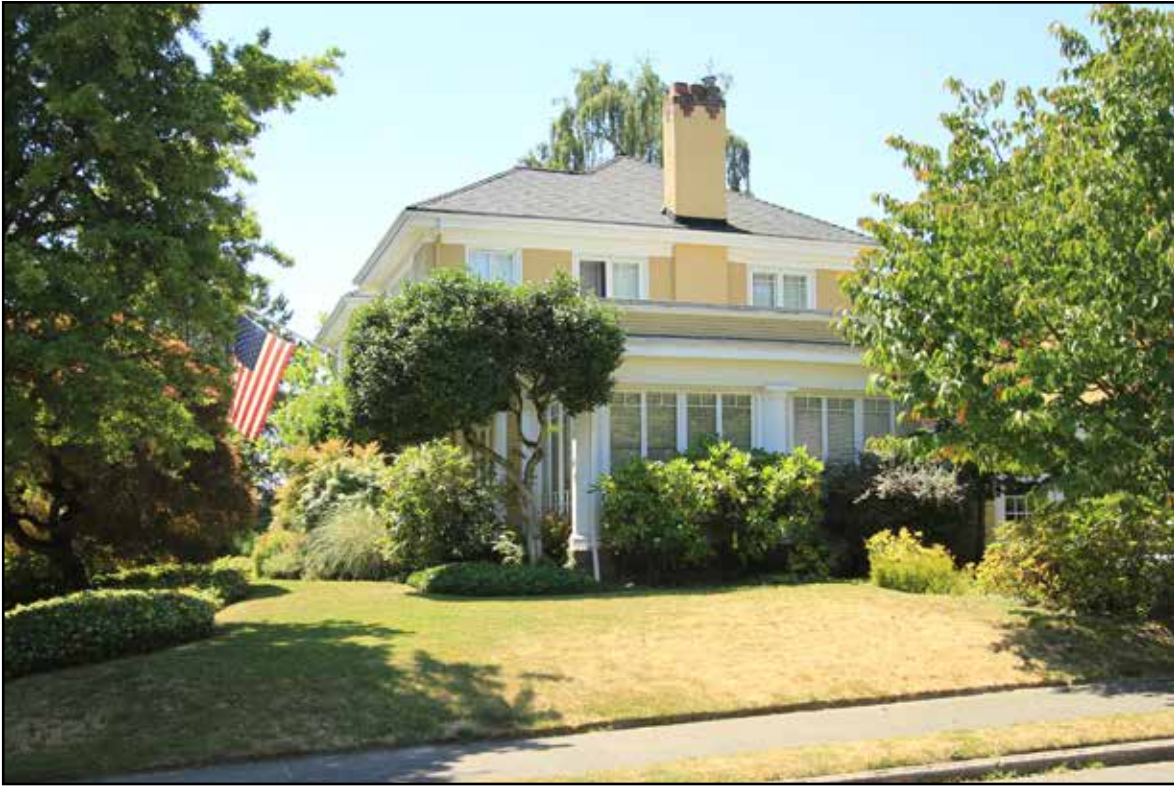
Fig 56. Frank Buty House, 3704 S. Ridgeway Pl. (1915; Charles Haynes, architect)
